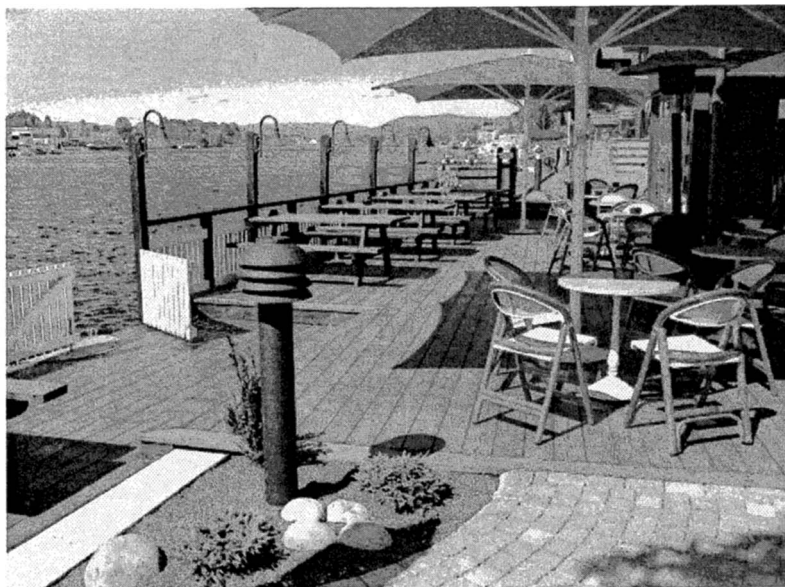
Figure 5. Decking of furfurylated Scots pine on a café in Porsgrunn Norway. Photo: WPT Norway
